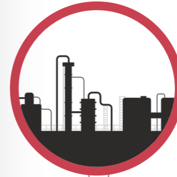
ONGC C2-C3 Extraction Plant
